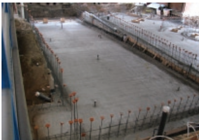
Top Left: Work begins in deep end of lap pool. Bottom Left: The floors of all three pools were poured in one day. Right: The concrete base for demising wall between new gymnasium from the weight room.
