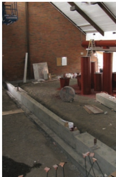
Top Left: Work begins in deep end of lap pool. Bottom Left: The floors of all three pools were poured in one day. Right: The concrete base for demising wall between new gymnasium from the weight room.
