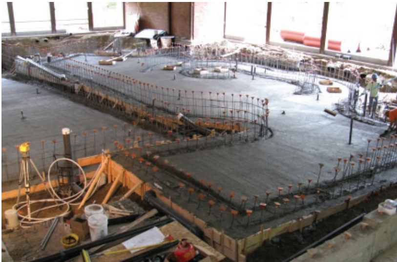
The concrete pool floors were poured on October 14.
