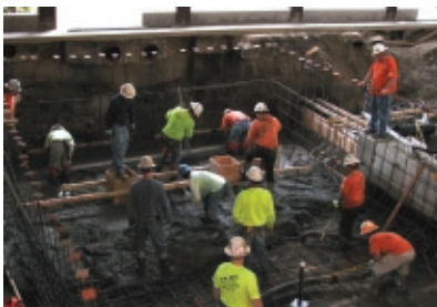
The concrete pool floors were poured on October 14.
