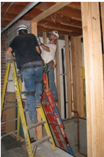
Left: Workers frame elevator shaft. Top right: Duct work system is installed on the natatorium ceiling. Bottom right: Concrete is poured on south end pool deck.
