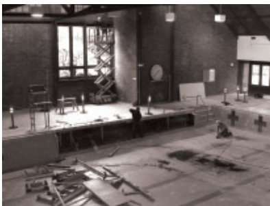
On May 13, 2009 crews began dismantling the aluminium pool shell.
