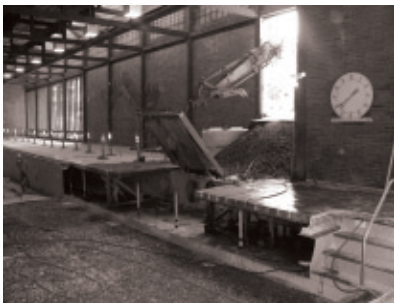
On May 15, 2009 crews began removing pool deck.
